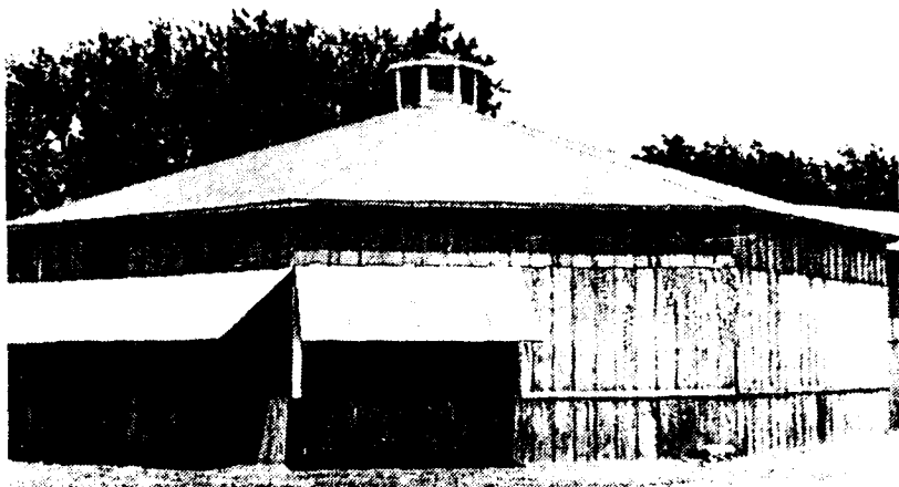
The building's design complements the carousel.
