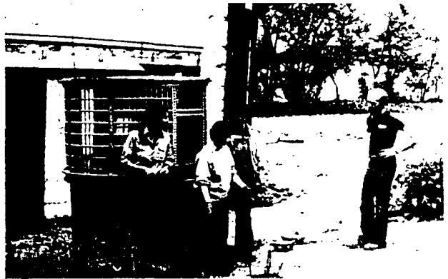
The ticket booth is a unique structure with a wooden lattice work top, a sheet metal bottom and a brass rail around the center. The rail matches the one on the Lovers' Tub on the carousel.
