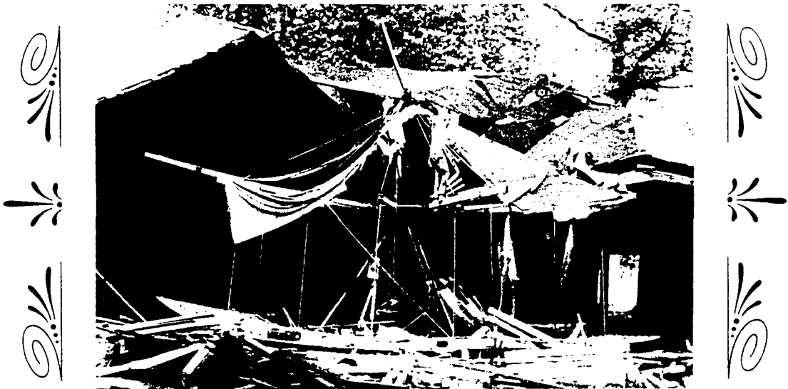
A disheartening sight greeted staff members of the Michigan State University Museum when they arrived in Crystal May 18, 1979 to begin disassembly of the carousel. The roof had collapsed under a heavy snowfall in January. The iron center pole of the carousel bore most of the weight and prevented extensive damage.
