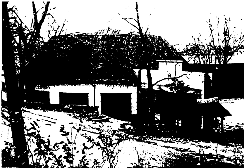
This fourteen-sided building was erected by a local carpenter when the carousel was moved to Crystal, Michigan in 1938. He set a telephone pole in the ground at the point where he wanted the center of the building and used it for support for the framework. When the building was completed he removed the pole and the building remained standing.
